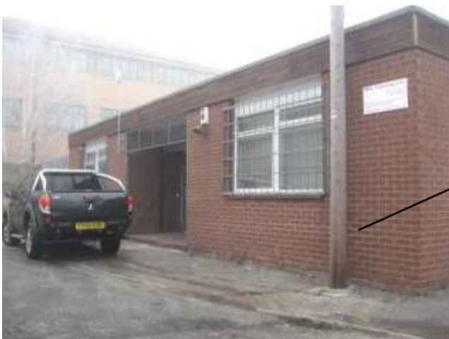
Electrical & Renewable Training Charlotte House 6 James Street, YORK
